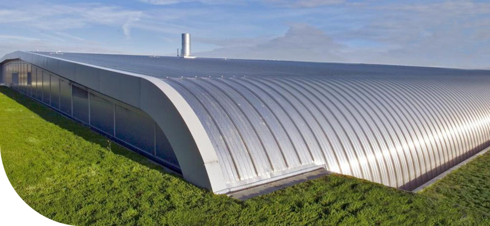
**Kalzip standing seam on Kalzip structural decking**
