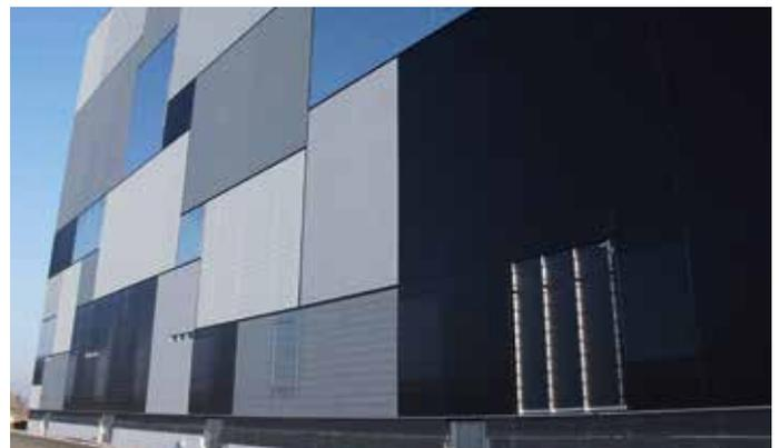
Direction-dependent installation of the Kalzip FC panels..
