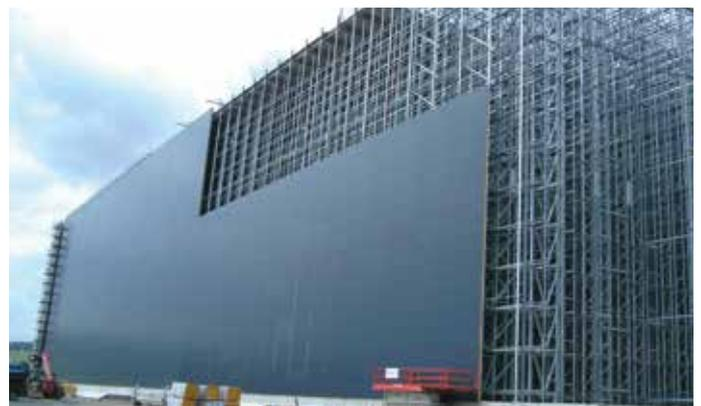
Fast economic installation of the FischerTHERM sandwich elements with DUO sealing.
