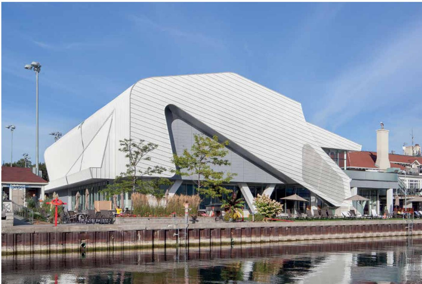
“We were really excited by the ability of Kalzip® to produce extremely long cladding sheets, each capable of being shaped to the precise profile of the building. This enabled us to design an elegant watertight structure able to withstand high wind loading and extreme temperatures whilst at the same time providing a clean, continuous and uninterrupted roofline that rolls seamlessly into the walls, creating a beautifully flowing building envelope.”
