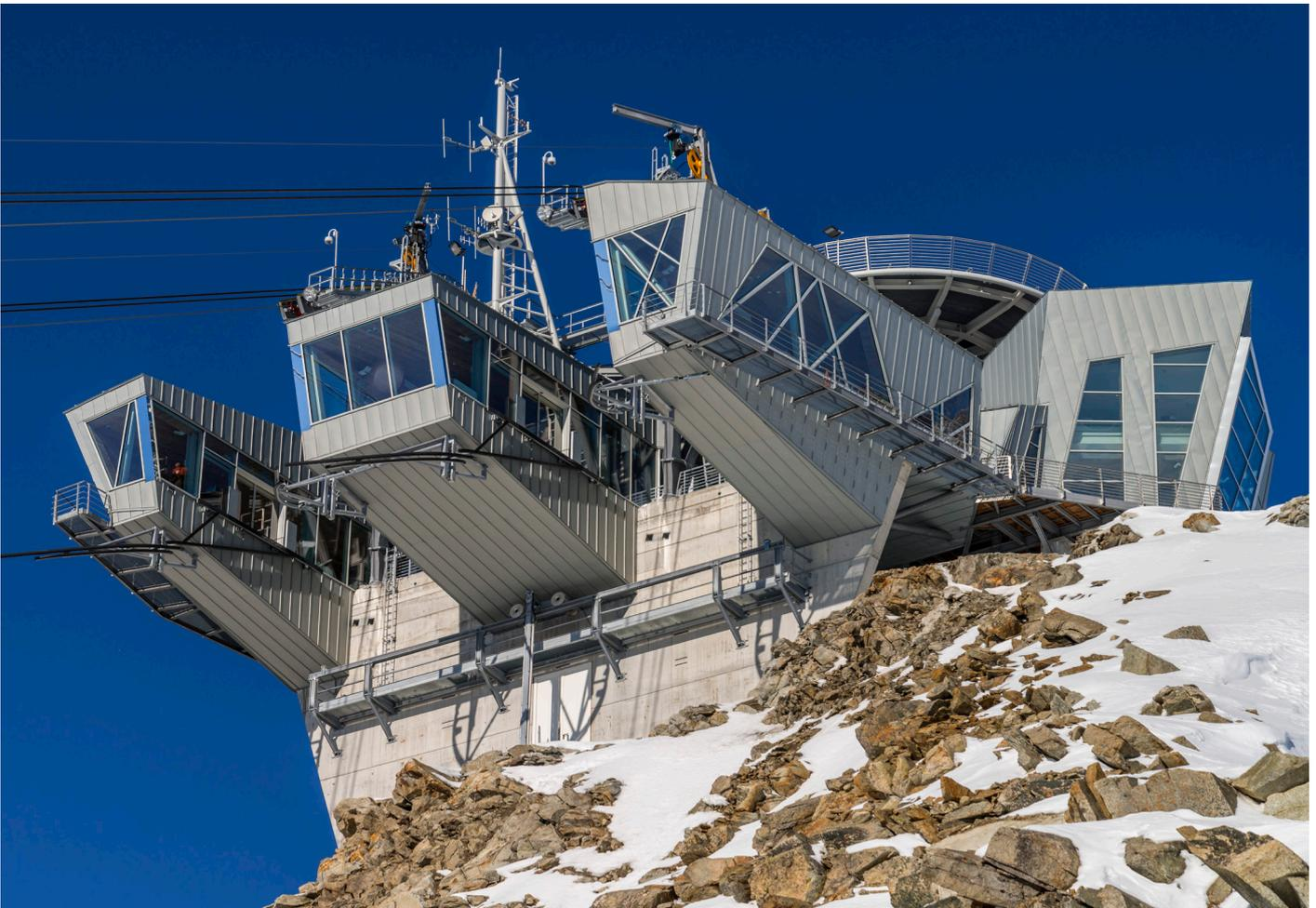
A Kalzip vapour control barrier was glued onto this. Finally, the visible exterior was finished in angled standing seam roofing, using 0.7 mm thick FalZinc® aluminium sheets. In total, around 7,000 m<sup>2</sup> of FalZinc® aluminium profiles were installed on the project.
