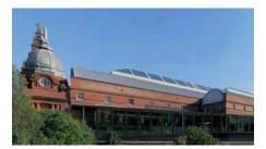
Manufactured inside the main hall, the Kalzip<sup>®</sup> sheets were then transported up to roof level for installation. The external face of the Kalzip<sup>®</sup> sheets has a highly durable AluPlusPatina finish providing a traditional appearance that blends sympathetically with the rest of the building and its surroundings.
