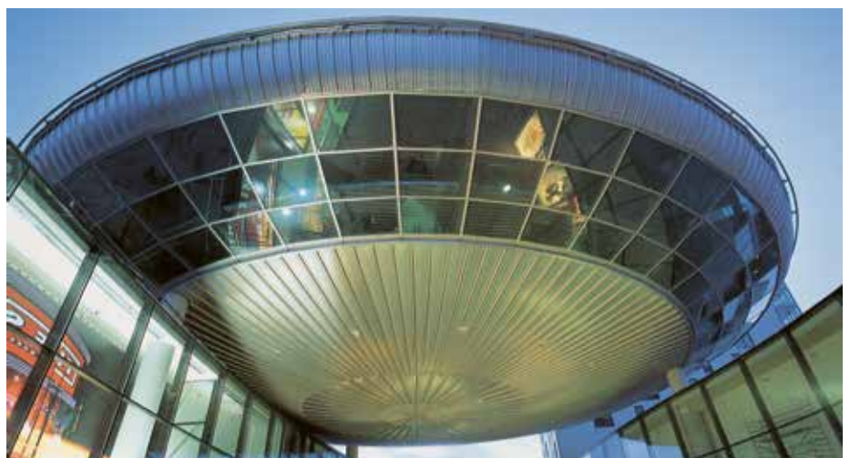
Spazio Zoetermeer (NL), Profile type 65/... tapered, stucco-embossed Architect: De Architekten Cie, Amsterdam
