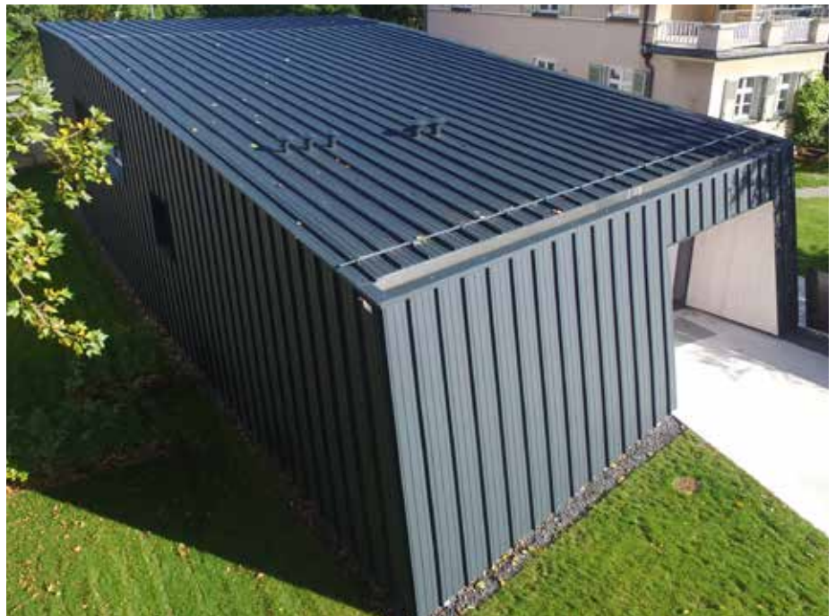
Martin Community Frankfurt-Schwanheim (DE) Profile type: 50/429, HPC 7016 3% Architect: Reuter + Werr Architekten BDA
