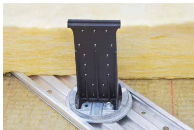
Swivel clip rail E with thermal insulation
