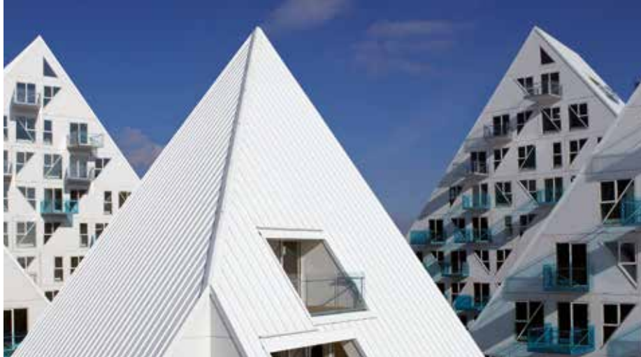
Residential complex The Iceberg (DK), Profile type: 50/400, RAL 9010 Architects: Cebra, JDS Architects, SeARCH and Louis Paillard
