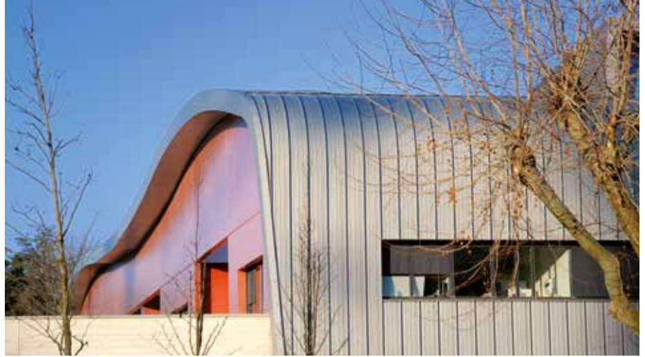
Biological Institute of the University Hospital Dijon (F) Profile type: 65/400, AluPlusZinc Architect: AIA Atelier de la Rize Architectes - Albert Constantin, Lyon
