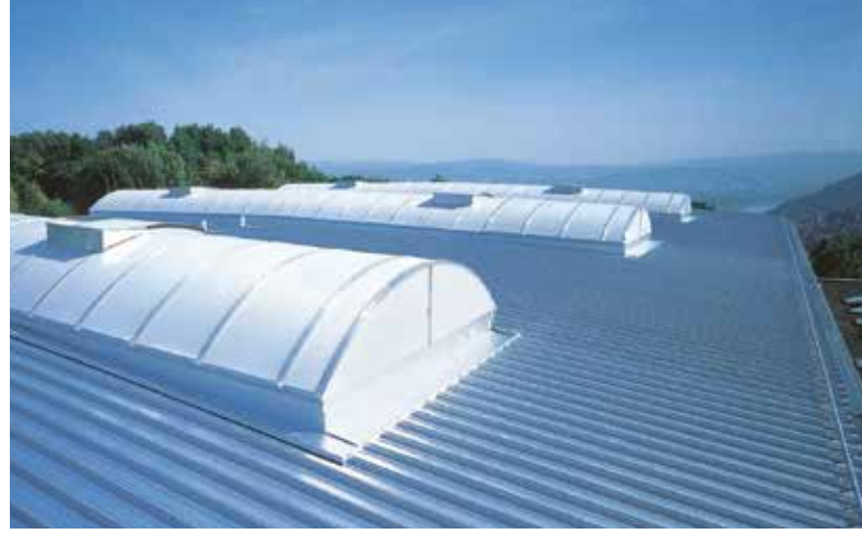
Vallendar comprehensive school (DE) before and after renovation; profile type: 50/429, stucco-embossed Architect: Guido Fries Architekten, Vallendar
