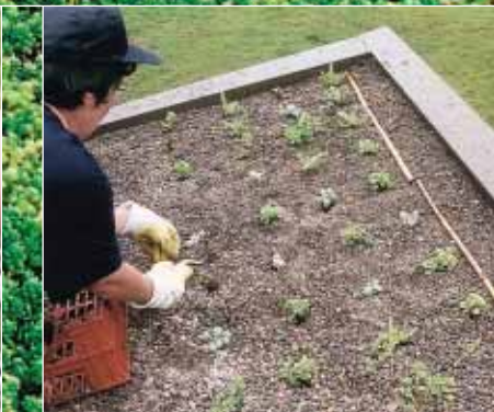
Planting out - a simple, rapid process. It takes a team of 3 just 2 hours to plant 3,000 plugs
