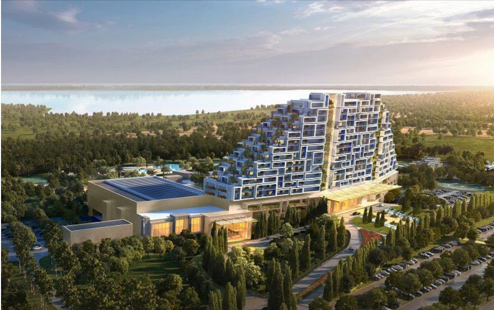
Back view of the building complex. The planned Kalzip roof is visible on the left-hand side
