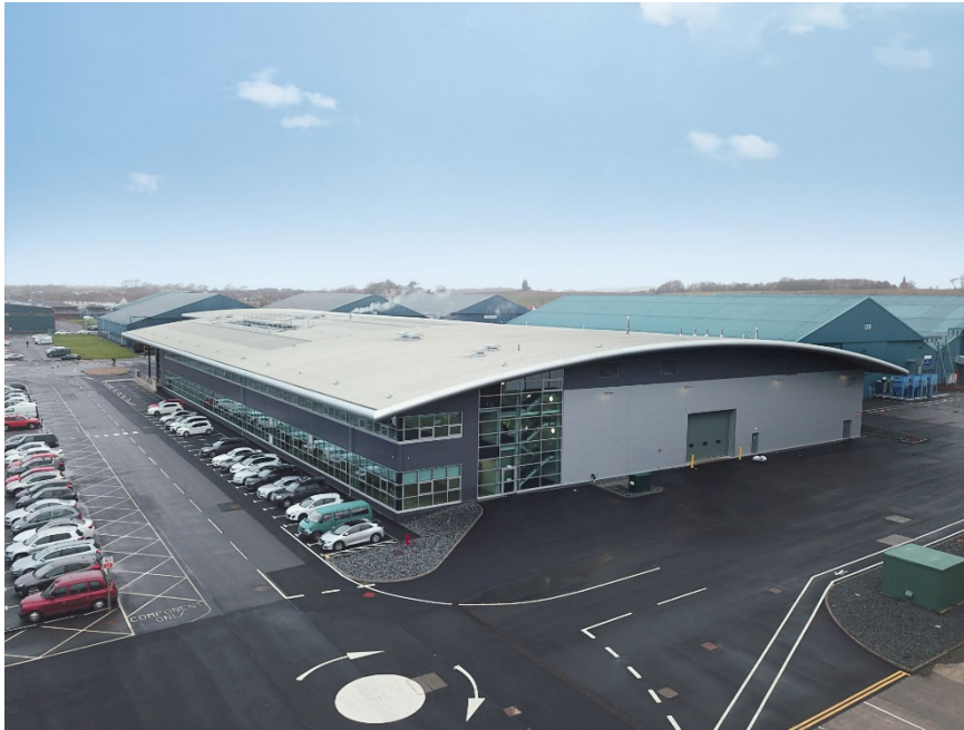
The bonded solution is streamlined to the roof and allows you to read the building form
